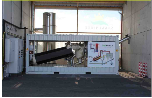
The charring is a pyreg reactor In the background is the exhaust heat exchanger
